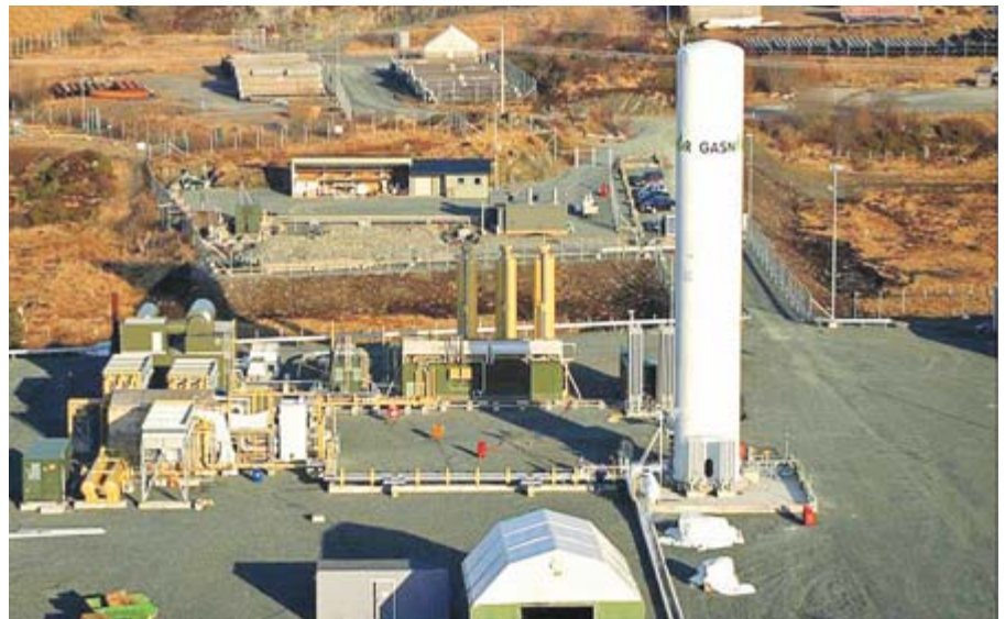
■ Fig. 1 - Small scale liquefaction plant at Snurrevarden, Norway.
