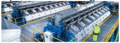
Wärtsilä's fast-starting internal combustion engine technology will be used to balance the power system and ensure its stability when the share of renewables is increased
