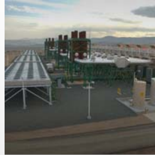
Grid stability and peaking
